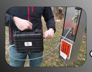
All Kupferle sampling stations are nondraining to avoid contamination of samples. With the use of our EEP (Electric Evacuation Pump) utilities can pump the unit dry to avoid freezing.
