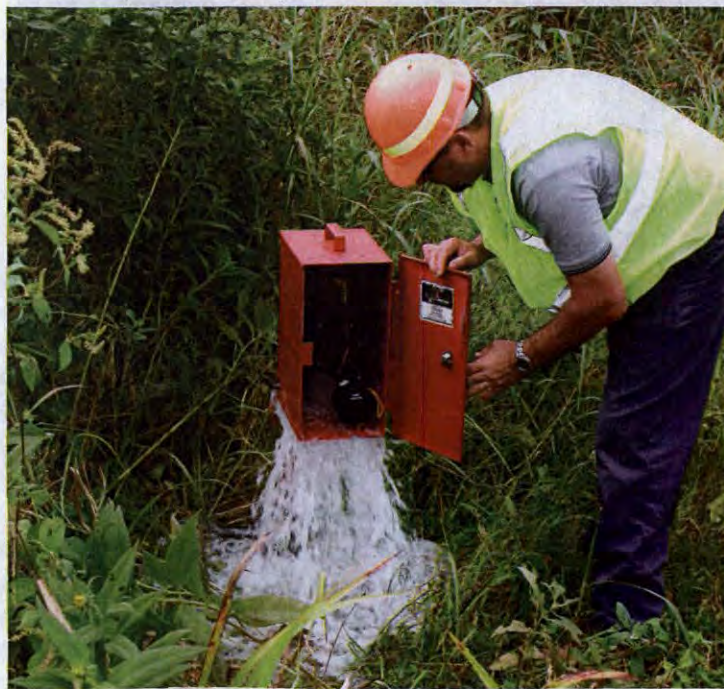
Mark Lee uses a portable automatic flusher from Kupferle Foundry.
