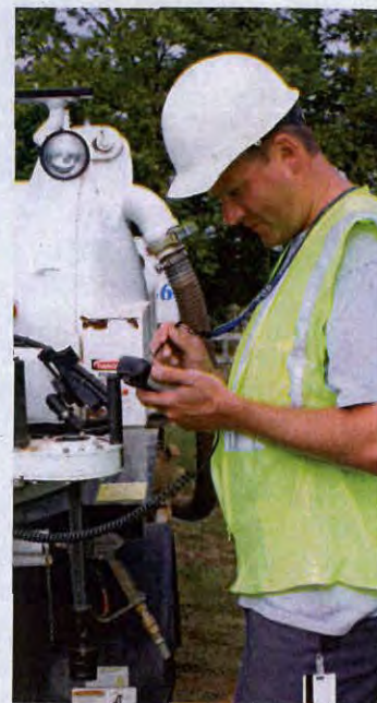
A PDA included with the valve maintenance trailer lets Glenn McCarty enter data on a valve.
