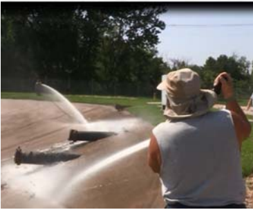
Plant workers cleaning retention basin using Kupferle's MainGuard #7500M Monitor Hydrants
