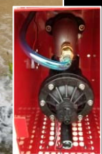
2" Solenoid Operated Valve (200 gpm max)
