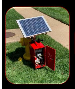
The 9250i's rechargeable 24 VDC lithiumion battery and wireless communications eliminate the rolling costs of site visits.
